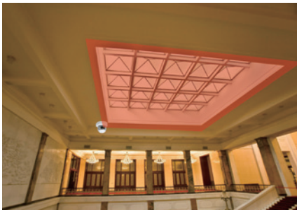
Skylight protection at Public facility / Warehouse
